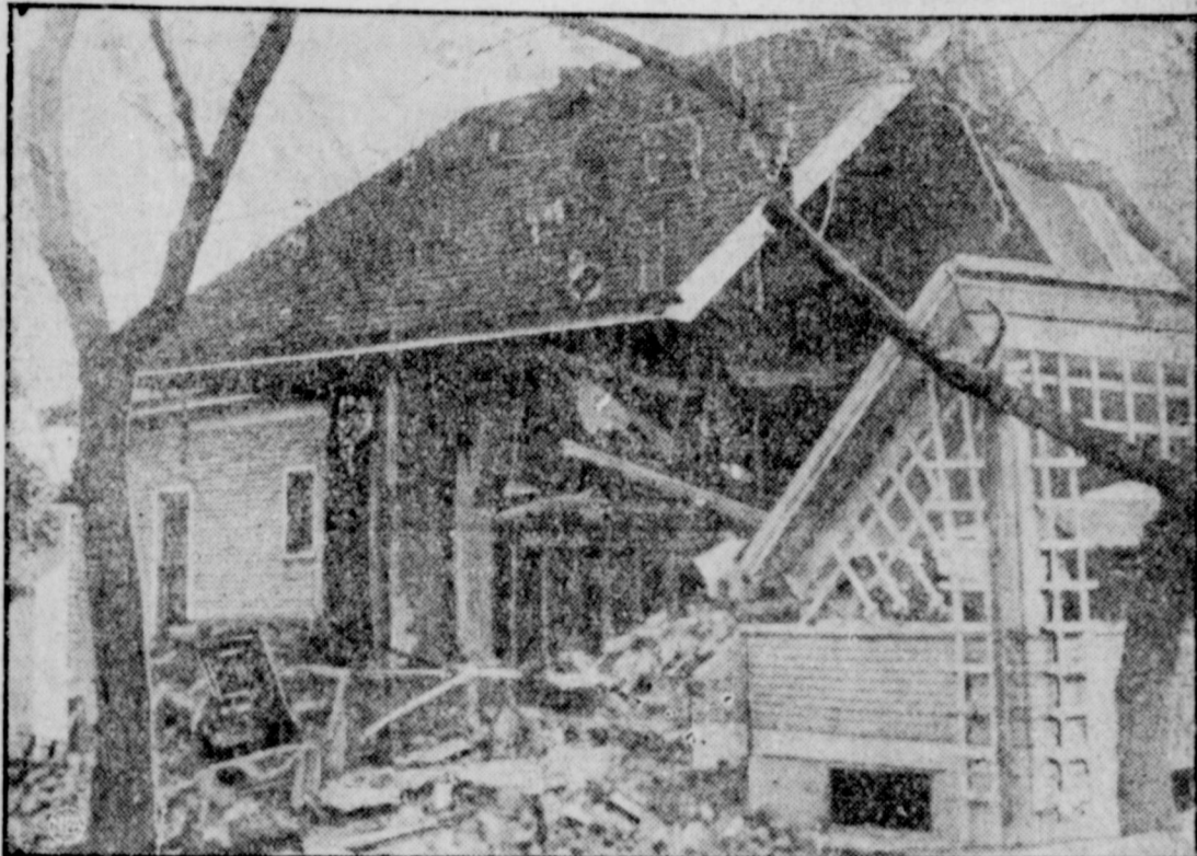
Typical of the ruin wrought by the quake which caused more than $2,000,000 damage and claimed two lives in Helena, Mont., is that shown at this home, where the occupants narrowly escaped with their lives when the structure collapsed. More than 400 buildings were damaged in the Montana capital, a city of 14,000, and the Red Cross has taken over the relief of scores of families. Hundreds of Helena residents fled in terror into the open country as shock followed shock.
