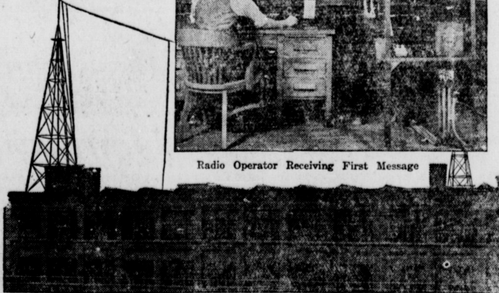
Aerial Atop Firestone Factory—Akron
