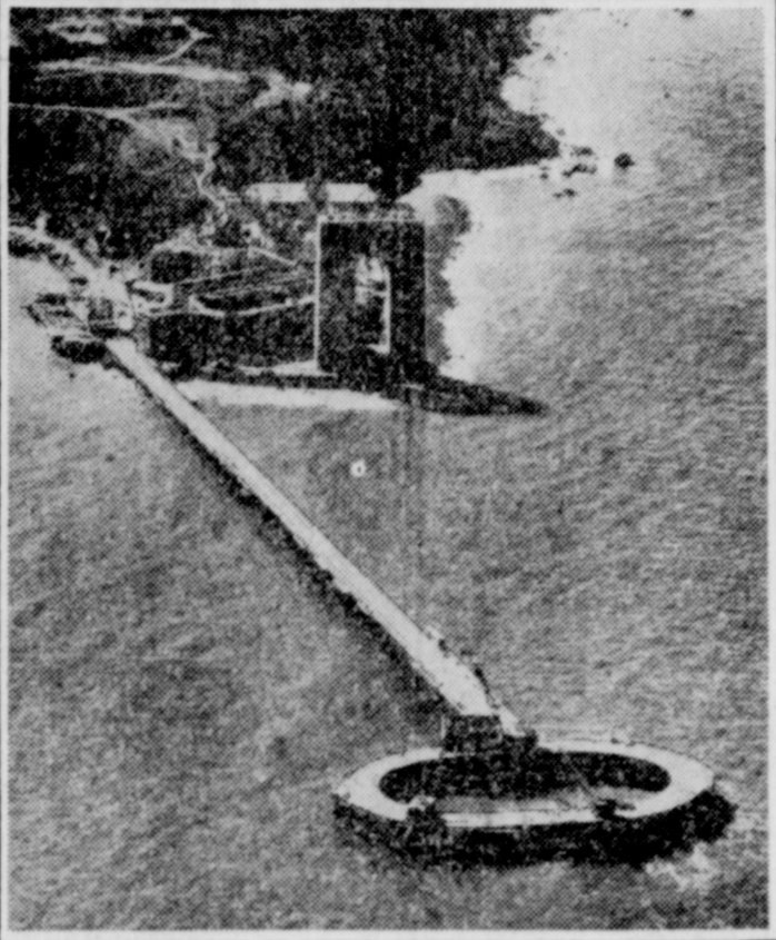
Seen from the air, the fender and trestle of the mammoth Golden Gate bridge, together with Fort Point, take the form of a gigantic key. A circle of concrete 750 feet in circumference and reaching 100 feet to the bottom of San Francisco bay forms a fender within which the south pier of the bridge will be built, protected from the tide-swept waters. The fender is seen lower right foreground in this picture, copyrighted by the Associated Oil Company.
