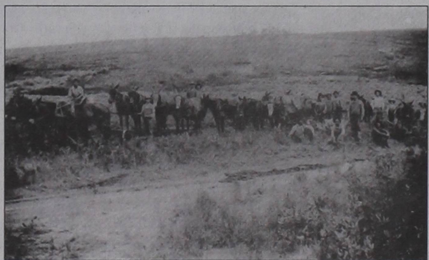
Friends and neighbors join the Tate family in this undated photo to help build two bridges on what is now County Road T, which are still in use on the Tate Place today.
