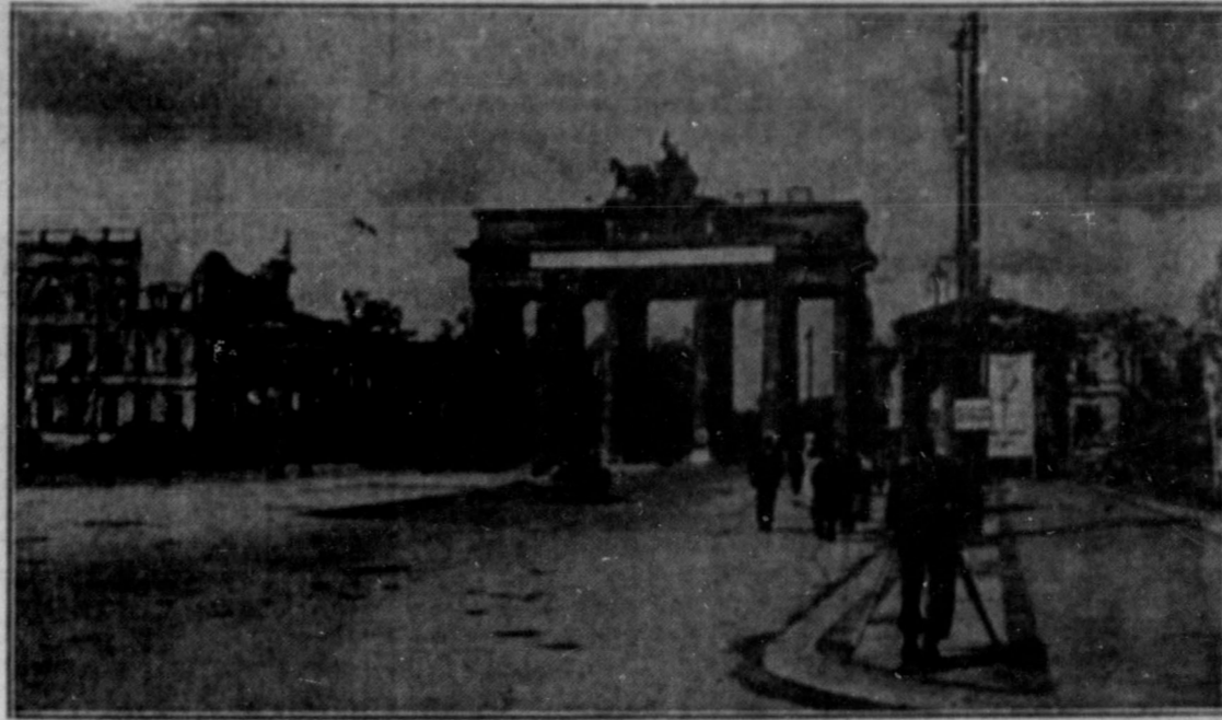
Released by U. S. War Department, Bureau of Public Relations. CENTER OF WAR-SCARRED BERLIN —The famous Brandenberger Tor in Unter den Linden still stands, but it was severely damaged by Allied bombs which demolished surrounding buildings.
