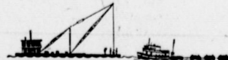
2,000-foot sections of pipe were shoved out into the lake, where tugs towed them to anchored barges.
