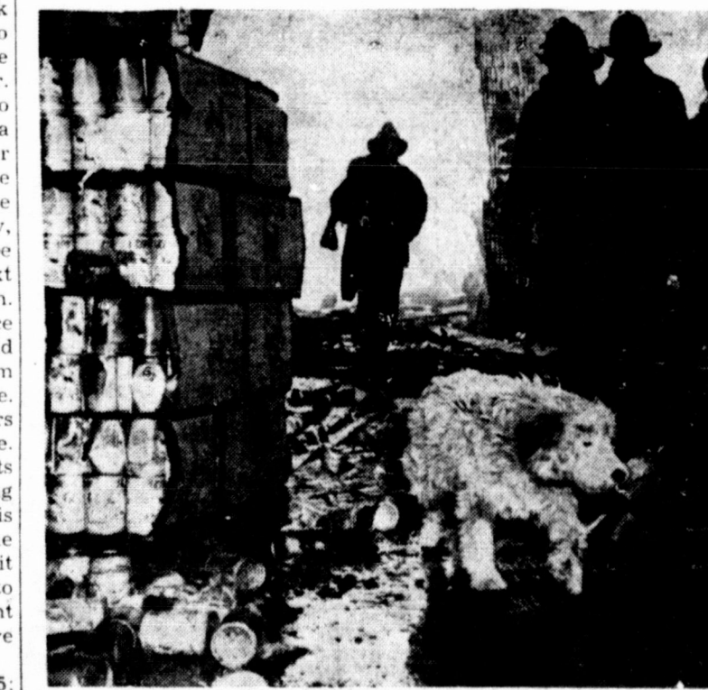
WHAT'S FOR DINNER? Weebegone pooch wanders through ruins of Los Angeles warehouse where fire destroyed $500,000 worth of dog food.
