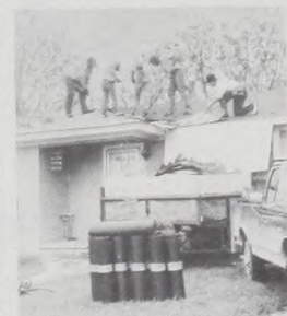
Fixing one of many hail-damaged roofs. JH
