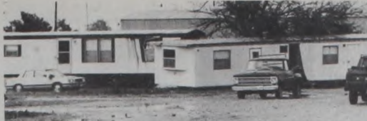
Flood-damaged trailer park. JH
