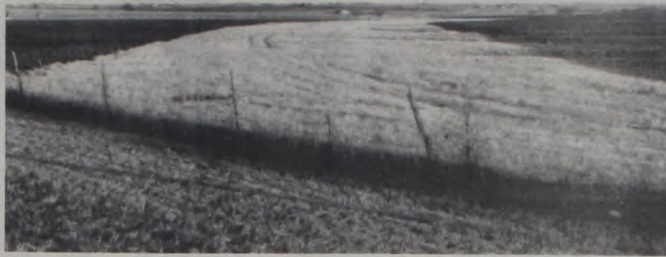
Established grassed waterway on Tony Trubenbach, Jr. farm near the intersection of FM-373 and FM-1630. The waterway serves as a safe outlet for parallel terraces to empty into.
