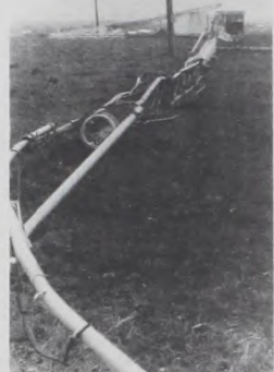
High winds crinkle Cooke Co. Electric Corp's radio tower.
