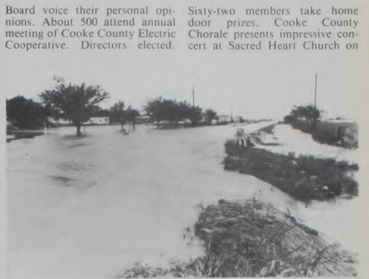
Heavy showers flooded Mesquite Street and other areas.
