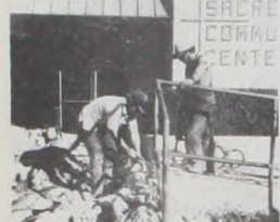
Workers reconstruct Community Center entrance.
