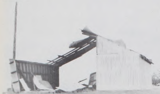
Local barn destroyed by high winds.
