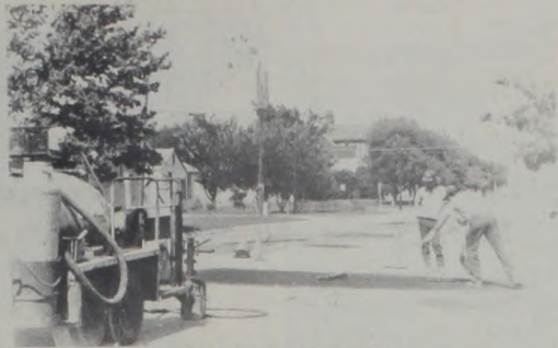
City workers repair Sixth Street.
