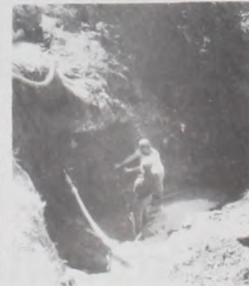
Workers in the hole, burying a line under the highway.
