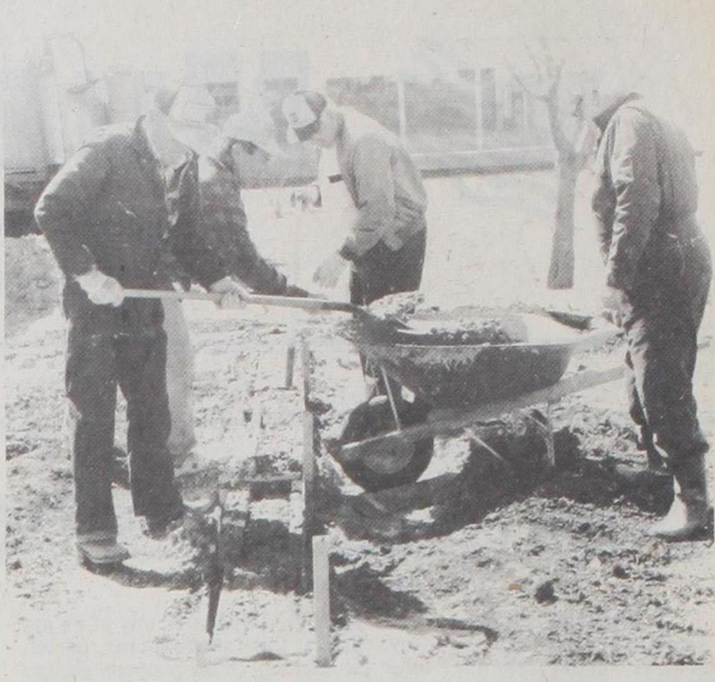
MUESTER KIWANIS CLUB members, l to r, John Rohmer, Butch Fisher, Wilfred Bindel and Vic Rohmer pour cement into forms to build the border edging for a large new flower bed in the Mid-Park, downtown Muenster. The flower bed will complement the new flagpole set up recently by the Kiwanians. Janie Hartman Photo
