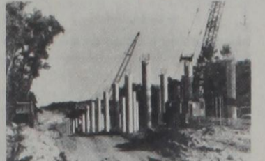
New Red River Bridge construction. jh
