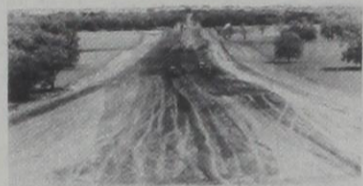
Work continues on Red River Bridge road. jh
