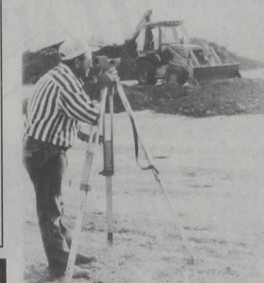
Construction begins on new Hornet gymnasium.
