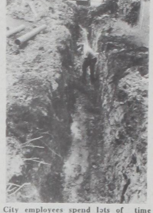
City employees spend lots of time repairing pipes. jh
