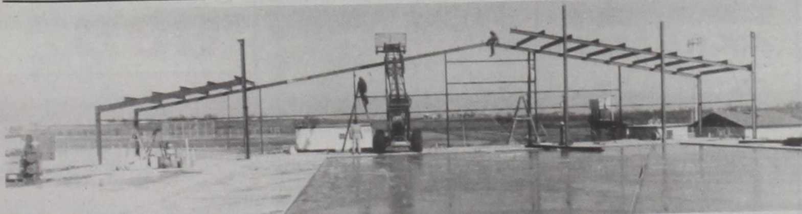
FRAMEWORK on Muenster ISD's new gymnasium appeared early this week as Structures, Inc. began the task of assembling the pieces together. Pictured above and at right are David Flusche and David Flusche Jr. and Shawn Flusche, connecting the steel beams on the north side of the building Wednesday morning.
