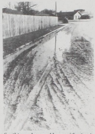
Southtown has problems with streets. jh
