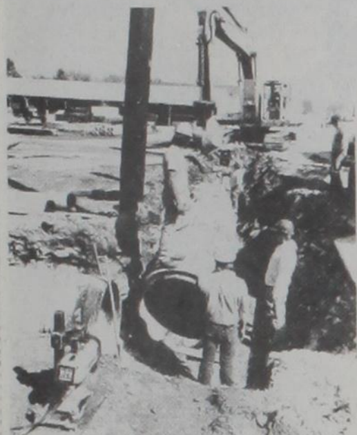
New drainage pipes installed on Main Street. jh
