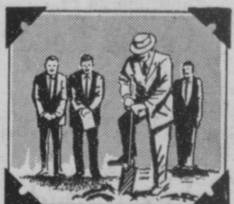
Broke ground for 2 new generating units with total capability of 740,000 kilowatts
