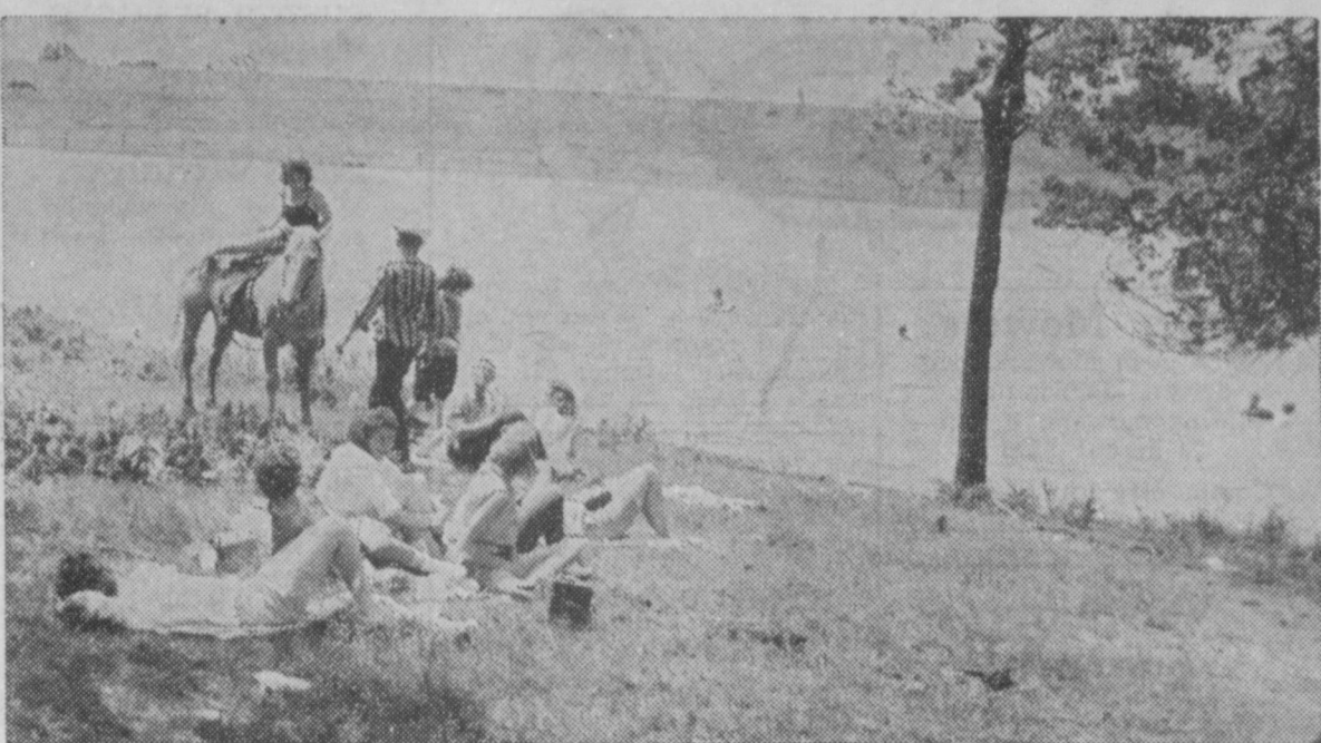
FLOOD PREVENTION structures like this one near Muenster bring fishing, boating, and picnicking to hundreds of area residents.
