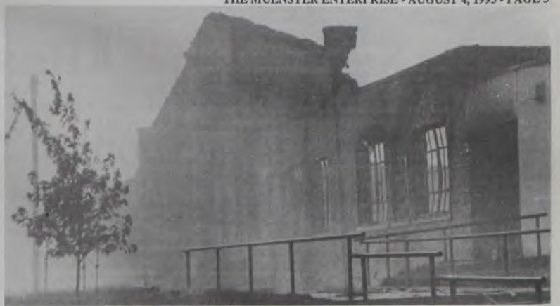
REMEMBER THE ALAMO? This Forestburg landmark reminded most area visitors of the Alamo. Fire gutted the school building early Wednesday morning, leaving the ghostly walls standing Wednesday as the debris continued to smolder.
