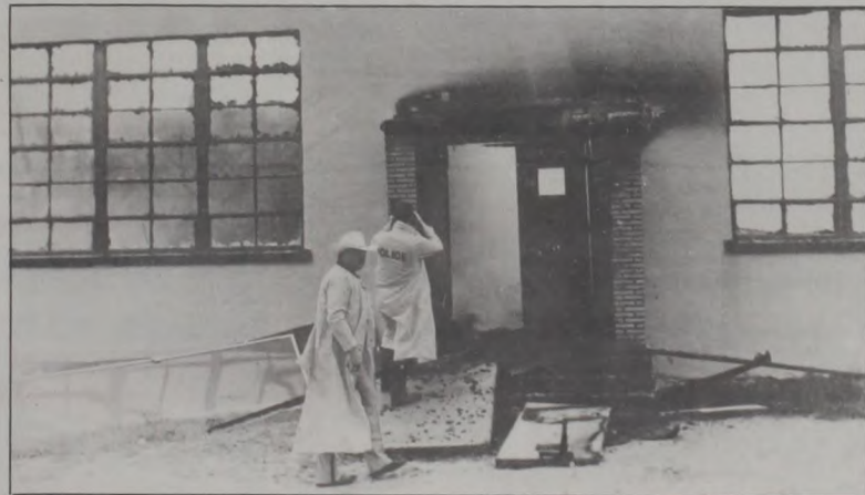
THE BURNING of the Forestburg School building lit up the skies early Wednesday morning as flames engulfed the gymnasium and classrooms, leaving only a smoldering shell on the hill at sunrise. Above, the Longhorns' gym (looking to the northwest) is now only a pile of rock and twisted metal. At left, Montague officers, including Craig Crawford with camera, photograph the outside of the building. This east door was blown out by interior explosions. Janie Hartman Photos
