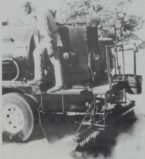
Resurfacing Oak Street was a relatively quick job Monday with major help from Cooke County Precinct Four. Above, Doug Yosten and Billy Poyner operate the gravel spreader. Below, Precinct Four Commissioner Virgil Hess operates the hot tar sprayer. The city pays for all materials. The county donates the use of the equipment. Dave Fette Photos
