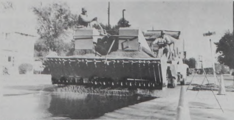
Resurfacing Oak Street was a relatively quick job Monday with major help from Cooke County Precinct Four. Above, Doug Yosten and Billy Poyner operate the gravel spreader. Below, Precinct Four Commissioner Virgil Hess operates the hot tar sprayer. The city pays for all materials. The county donates the use of the equipment. Dave Fette Photos
