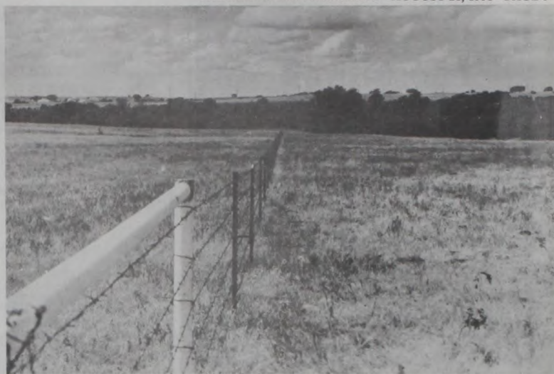
This fence row marks the approximate location of the dam that will hold the water to create Muenster Lake. The wall of dirt will be about a mile long, stretching southwest through the bottom land to the bluff near Highway 82. Construction is scheduled to start in July 2000. Photo by Janie Hartman
