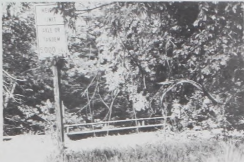
Eddy Street bridge closed.
