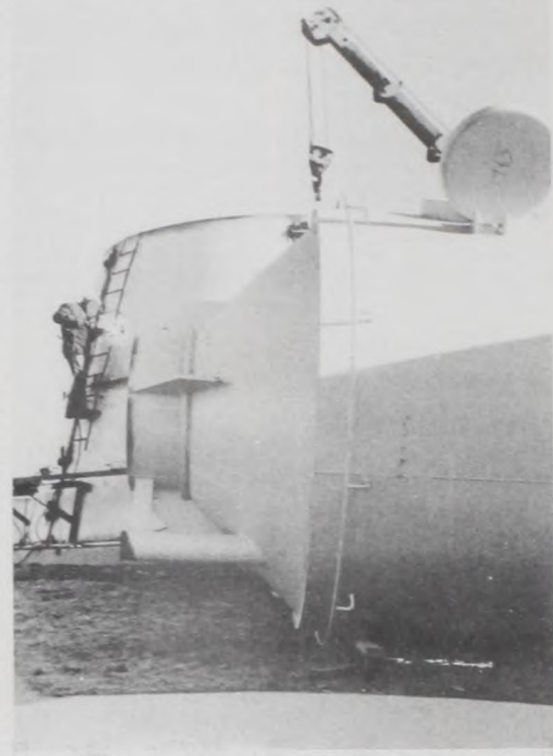
Building a 200,000 gallon water tank.
