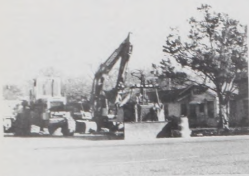
Twelve inch water line installed.
