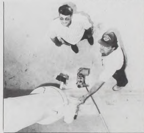
Inside the new water tower. DF
