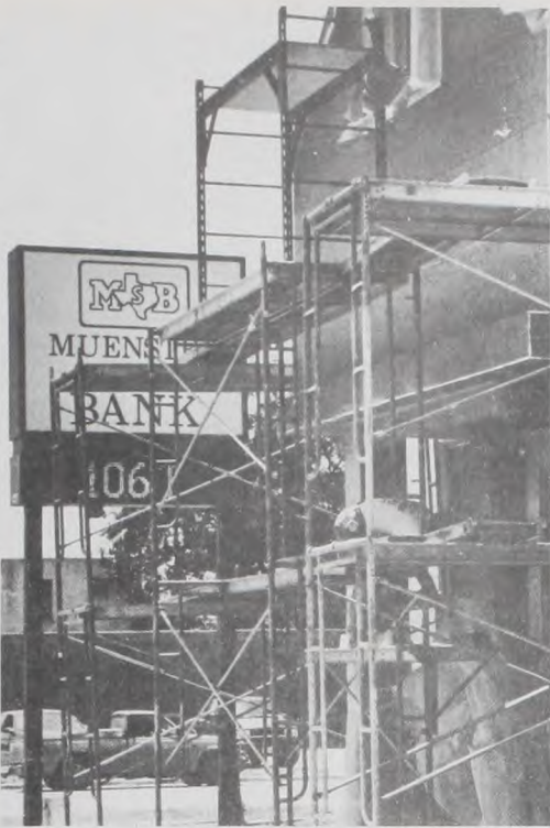
Hot days — bank construction.
