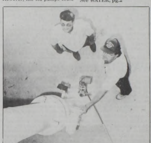
Steve Broyles and Chris Yosten make adjustments inside the base of the new water tower. Photo by Dave Fette
