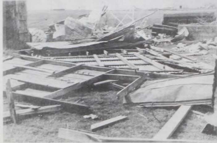
High winds last weekend are blamed for the destruction of a garage/shed located on the old Trubenbach farm south of Muenster. The straight winds leveled the building, spreading tin, lumber and other debris in a north easterly line through the barn yard.
