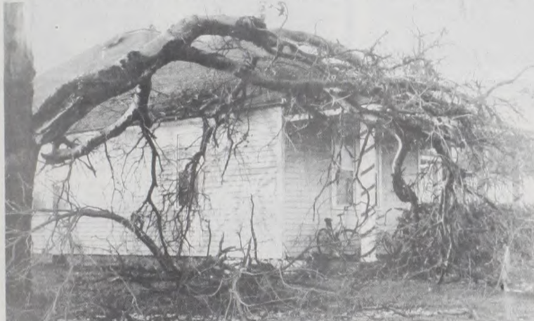
The home of Cathy and Francis Fuhrmann on Oak Street in Muenster received minor damage when a neighboring tree fell during the holiday ice storm. Janie Hartman photo
