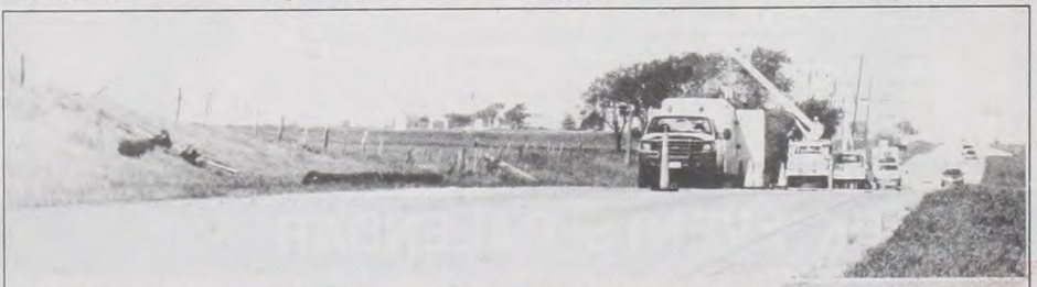
TXU Electric transmission and distribution crews lined the east bound lane of Hwy. 82, near Myra all day Wednesday repairing lines and re-installing seven poles that were broken off by high winds around 2:30 a.m. Wednesday. Electricity was off in the cities of Muenster and Myra. Muenster was back on at 5 a.m., receiving power from the west and Myra was out until 7 a.m., getting back feed from Lindsay. Photo by Janie Hartman
