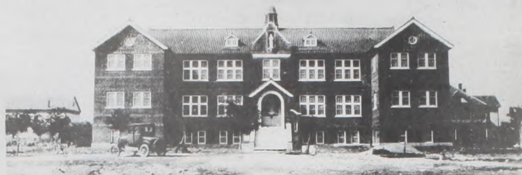
Sacred Heart School shortly after completion in 1924. To the left is the parish hall and to the right the convent, now part of the "tin university"
