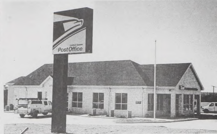
Progress continues on the completion of Muenster's new post office
