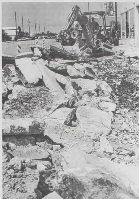
Curb work begins, kicking off the KMB beautification project
