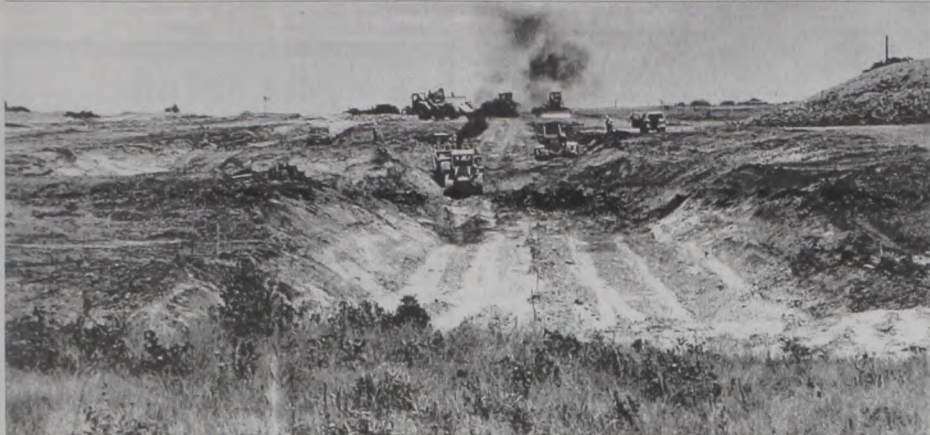
Work is progressing at the site of Muenster Lake as equipment digs out the "back drain" of the dam. The drain, 40-foot wide at the bottom located on the backside of the dam, will take care of any future seepage. Below - Heavy equipment works on the
