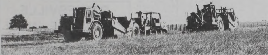
Work is progressing at the site of Muenster Lake as equipment digs out the "back drain" of the dam. The drain, 40-foot wide at the bottom located on the backside of the dam, will take care of any future seepage. Below - Heavy equipment works on the
