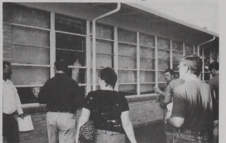
Lindsay ISD Superintendent Travis Winn conducted a walk-through inspection of deficiency items listed by the Lindsay School Board. All problem areas that needed repairing, cleaning or painting were completed to the Board's satisfaction on schedule. More problem areas are due for inspection on Aug. 11. Dave Fette Photo
