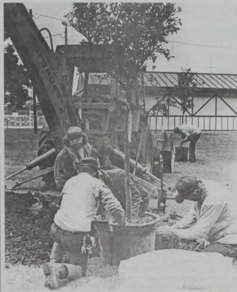
Muenster city employees planted six trees in the City Park this week as part of the Keep Muenster Beautiful and Tree City Beautiful organized effort. The trees are Bur Oaks and Cedar Elms and were planted in the opened area south of the pool complex. Janie Hartman Photo
