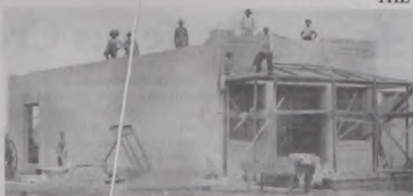
Sisters: the "Gehrig" building being built in 1909-10.
