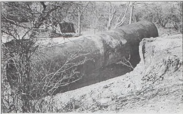
A new culvert, above, falls into the opening after the County Precinct #3 crew "pushed" it with equipment. The drain "pipe" was placed next to the original concrete bridge wall, on the east side of the ditch, built before 1923. Below, the workers discovered four names and an initial on the wall of the old bridge. Names found were F. Becker, V. Hartman, F. Klement, and J. Hesse. The guys wrote their names in the wet cement over 80 years ago. (Names were enhanced on photo to improve visibility.) Janie Hartman photos
