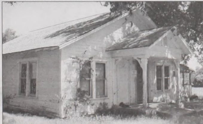
Part of Cooke County's history no longer exists. The manager's house (above), the Poor House, and several other buildings were dozed last week.
