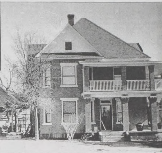
garage/shop addition gets covered. The inset picture shows the back (east) side of the project. Janie Hartman photo
