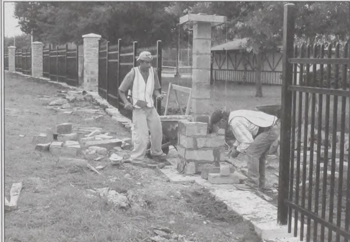
Rain-delayed work continues on the Keep Muenster Beautiful project being constructed at the City Park along Highway 82. Muenster won the 2004 Keep Texas Beautiful Governors Award of approximately $65,000 to fund the project. The 700 foot decorative wrought iron fence with stone masonry columns went over budget. The City donated extra rocks left over from the entry, and TxDOT covered the remaining cost to finish the job. KMB is attempting to win the award again this year. Janie Hartman photo
