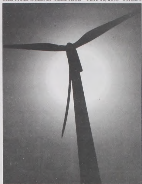
A recently assembled wind turbine generator (WTG) turns very slowly in the wind, but will not generate energy until this fall. It is one of the first to be assembled at Wolf Ridge Wind, L.L.C. located north of Muenster. Each blade is 132.2 feet long and weighs 13,338 pounds. Janet Felderhoff photo
