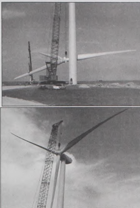
A recently assembled wind turbine generator (WTG) turns very slowly in the wind, but will not generate energy until this fall. It is one of the first to be assembled at Wolf Ridge Wind, L.L.C. located north of Muenster. Each blade is 132.2 feet long and weighs 13,338 pounds. Janet Felderhoff photo
