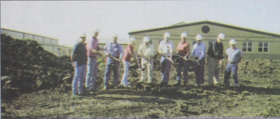
Muenster ISD officially broke ground last week on the construction of a new cafetorium and classrooms project. Pictured are, from left, Bill Krieger, building project superintendent, Board members Mel Walterscheid and Neal Flusche, Elementary Principal Lou Heers, Board members Jeff McAden, Ronnie Felderhoff, and Steve Trubenbach, Rudy Koesler's building committee member, John Kaufman, MISD superintendent, and Kirk Dawson, project manager. Not pictured are Board members Bert Walterscheid and Jim Endres. Janie Hartman photo
