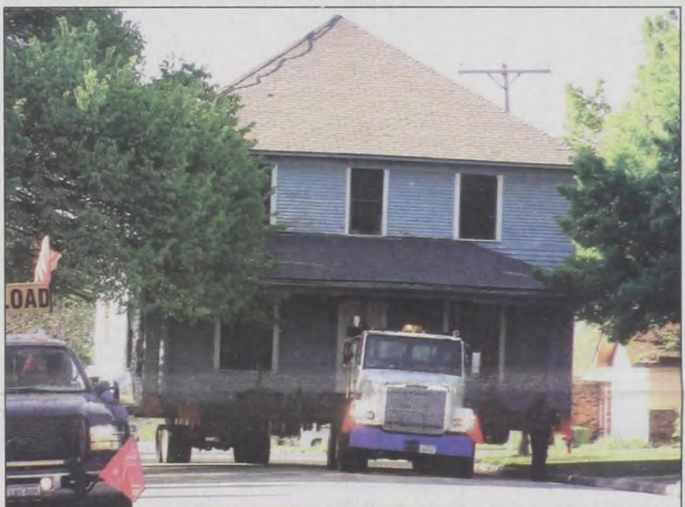
Muenster's tree-lined streets were just a few of several obstacles encountered Monday when the Lehnertz house traveled through town to its new home. See inside for more on the move. Janie Hartman photo
