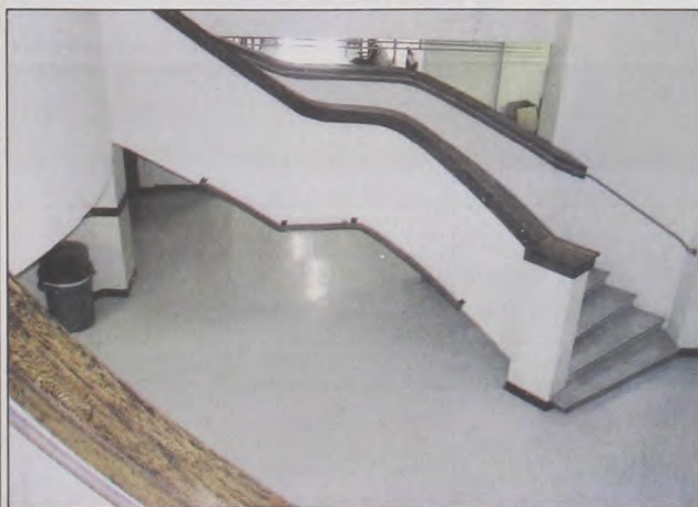
Cooke County's Courthouse has many empty offices and few visitors these days. The hustle and bustle of routine County business no longer takes place in the Courthouse. Most offices with their county officials and employees have already moved to their temporary locations. They will remain outside of the Courthouse until the facility is restored to historically correct state. The restoration is being partially funded through grant money received to restore Texas courthouses to their original condition.
