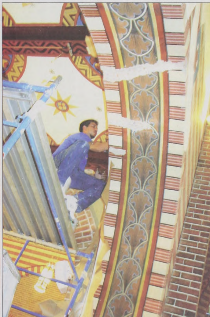
What started as filling cracks in the walls and a repainting job, has turned into a big mess in St. Peter's Catholic Church in Lindsay. Major water damage was found, which is now being replastered and painted. Darrell Mayo of Plano and his crew of nine or 10 workers will also restore some of the art
