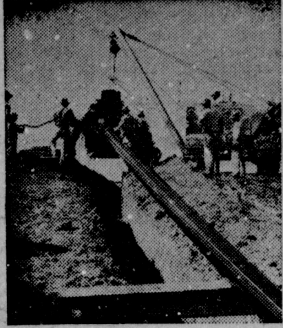
The output of Humble Oil & Refining Company's big Baytown plant was brought closer to the gasoline-consuming public of North Texas last Tuesday, October 15, with the formal opening of the Dallas-Ft. Worth terminal and distribution center. This terminal will serve the area within a radius of 75 miles or more with gasoline delivered through the 275-mile eight-inch line shown under construction in this picture.
