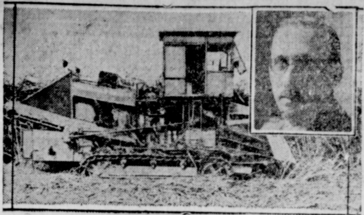
Cutting an acre of sugar cane an hour, equalling about 150 hands, a new harvester has been set to work near Clewiston, Fla. The harvester, shown here, is the work of Carl G. Muench, in inset, of the Dahlgren Sugar Cane Industries. Working three eight-hour shifts a day, it will cut more than 480 tons of cane.
