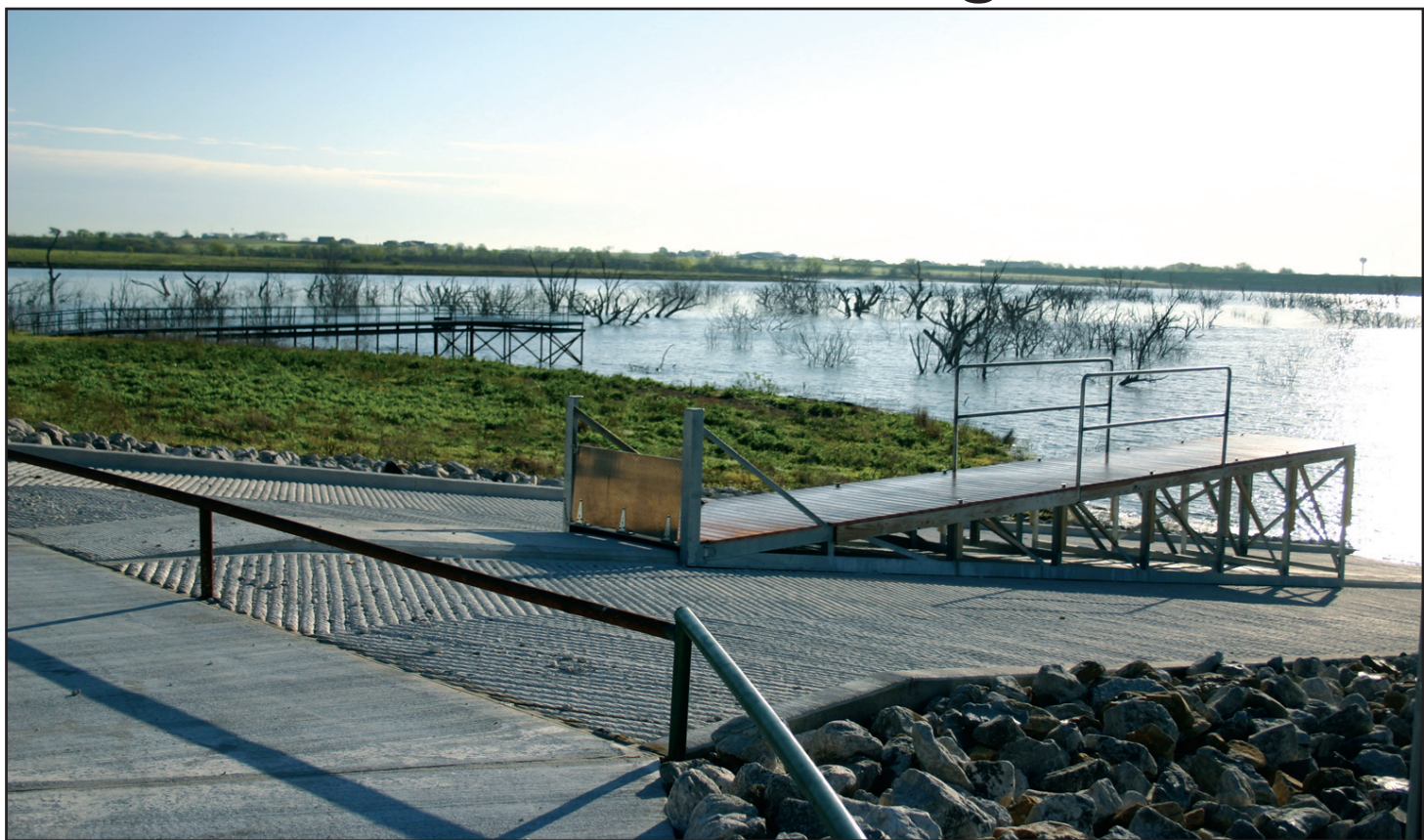
Sunny Spring weather returned Wednesday morning after a swarm of thundershowers dumped anywhere from two to more than three inches of rain on the area. With rain falling for over 24 hours, water runoff into Muenster Lake has contributed to a noticeable rise in the water level, but much more rain is needed to "fill" the Lake. Janie Hartman photo
