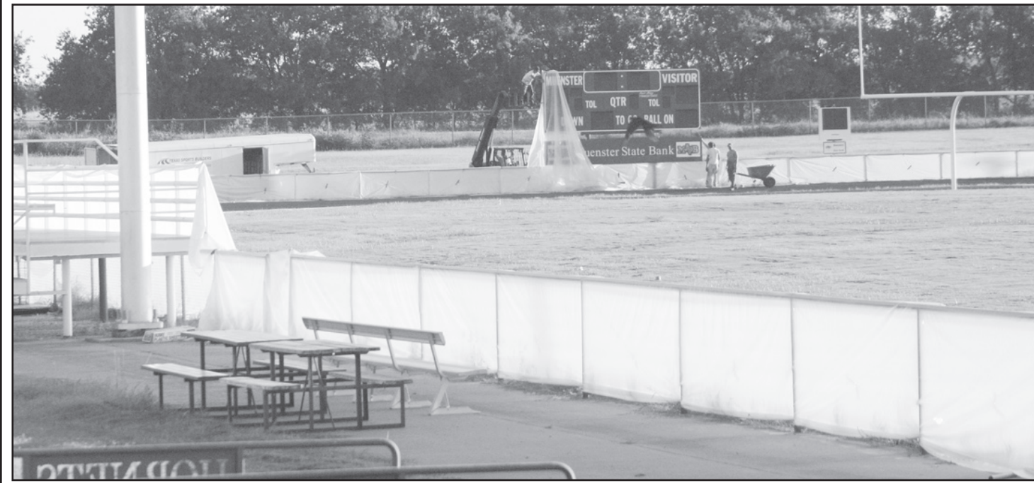
Workers hung plastic on the fence and other areas around the Muenster Hornet football field this week for protection in preparation of spraying a new surface on the track.
