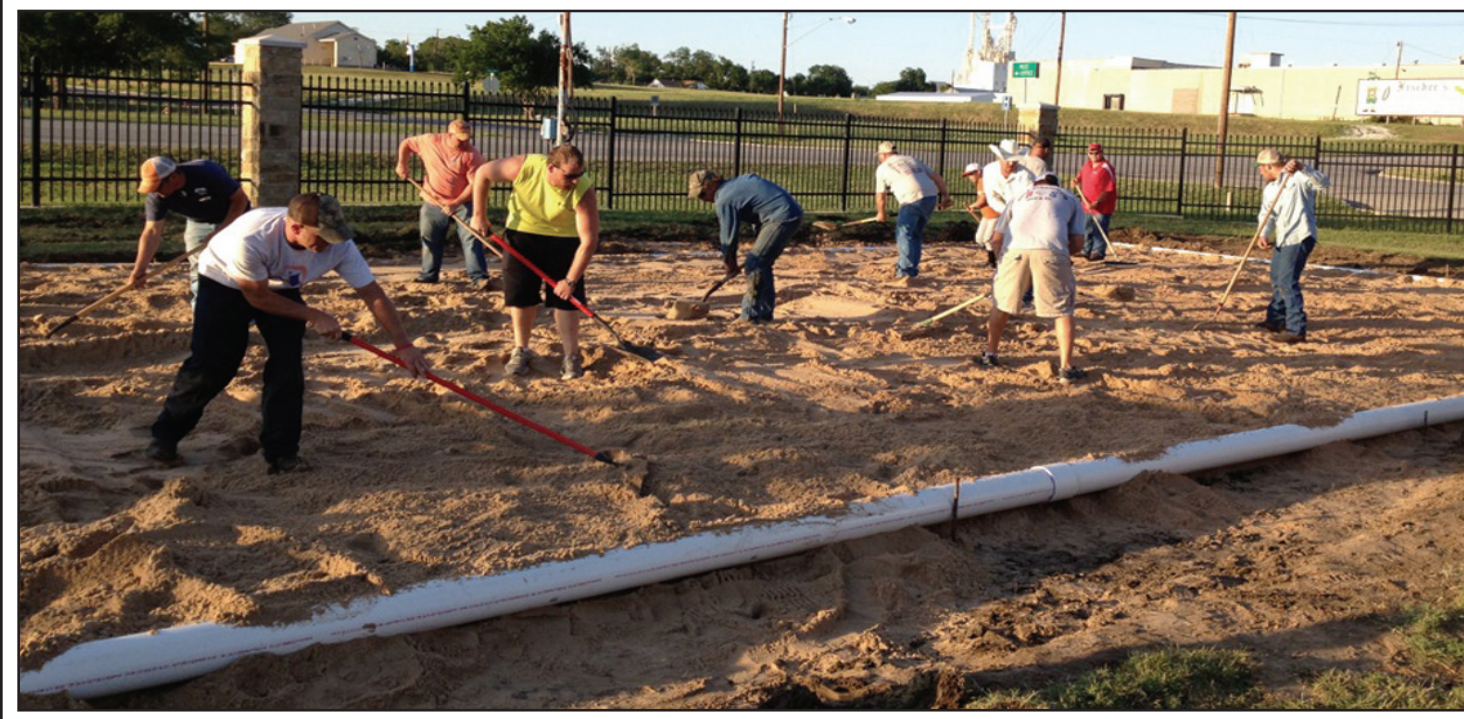
Muenster Jaycee members were busy in the City Park last Thursday and Friday refurbishing the sand volleyball court. Work consisted of digging out the old sand, grass, and stickers. They put in wash sand from east Oklahoma, new dirt around the edges, put up a new net, and fixed a broken light. The boundaries are now constructed of 6" pvc pipe. Alan Ritchey donated two loads of sand and G&H Backhoe and Dangelmayr Construction donated the use of their equipment for the project. Courtesy photo
