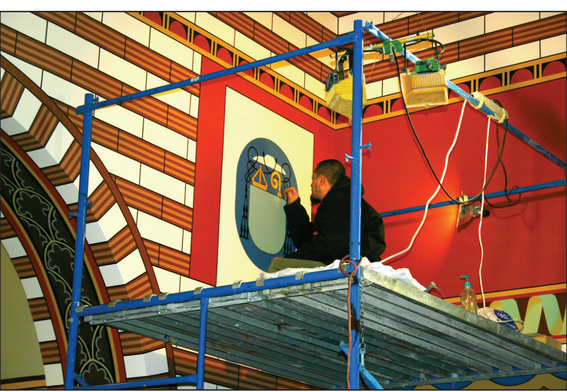
Work continues inside St. Peter's Church. Above - a painter replaces art that was lost in the crumbling plaster; below left - an area with all plaster removed; below right - redrawing the design in the Baptismal room.
