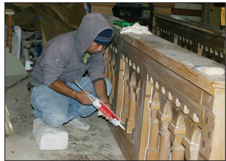
Repairs go beyond plaster and painting the walls.
