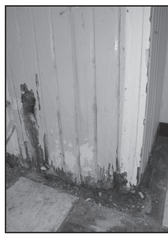
The old practice gym (built in 1949) has safety issues: the floor has sunk over six inches in some areas; there is termite and water damage. The practice gym is necessary to allow all ten school teams time to practice.
