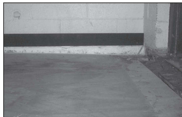
The old practice gym (built in 1949) has safety issues: the floor has sunk over six inches in some areas; there is termite and water damage. The practice gym is necessary to allow all ten school teams time to practice.
