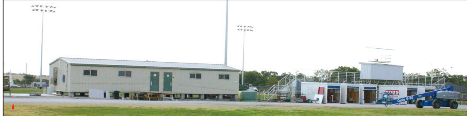
Storm damage to the Tiger field house and weight room forced Sacred Heart to move in a portable building and containers for storage, until a new den can be built. Janie Hartman photo
