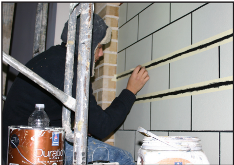
Redrawing and repainting designs on the walls covered by plaster repair
