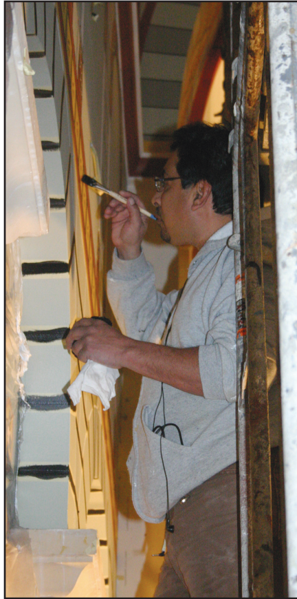
Redrawing and repainting designs on the walls covered by plaster repair
