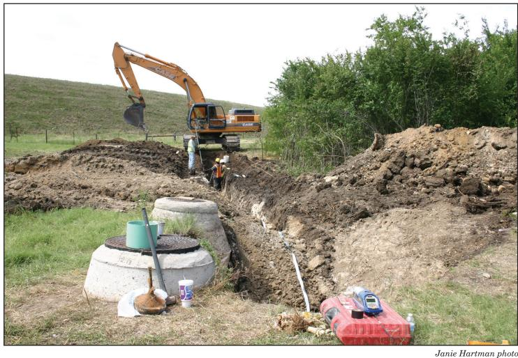
Work continues on replacing a 1950 sewer line that lays under Weinzapfel Lake dam. Unable to get permission to bore under the dam, the City must reroute the drainage line around the east side of the dam before major problems start to occur. Pictured, work began on the southeast side of the dam.
