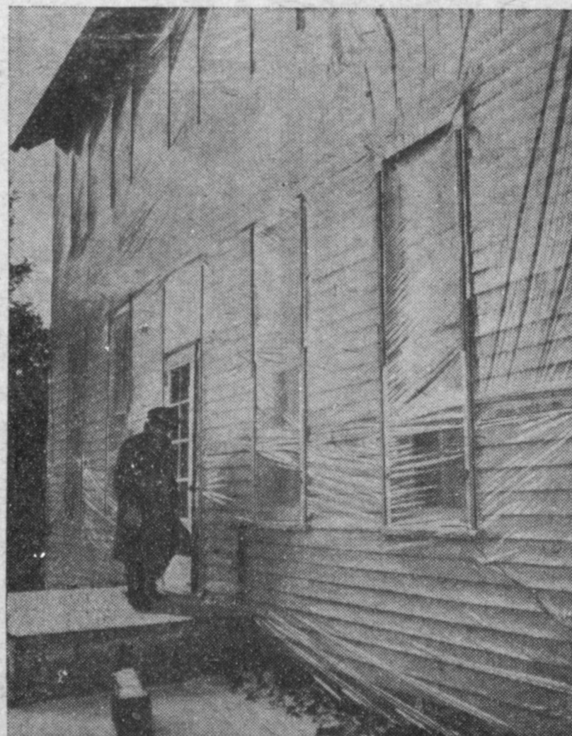
WRAPPED FOR WINTER—Wrapped in shimmering polyethylene, this old house in Lafayette, Ind., is the result of one cold winter night when the temperature fell to 10 degrees below zero. The goldfish bowl in the living room froze over, despite the fact that the oil burner was on. Purdue University Agricultural Experiment Station suggested wrapping the poorly insulated building in polyethylene film. Agricultural engineers are still testing the temperatures inside and out, but the residents of the house have been able to turn down the oil burner at night, even in coldest weather.
