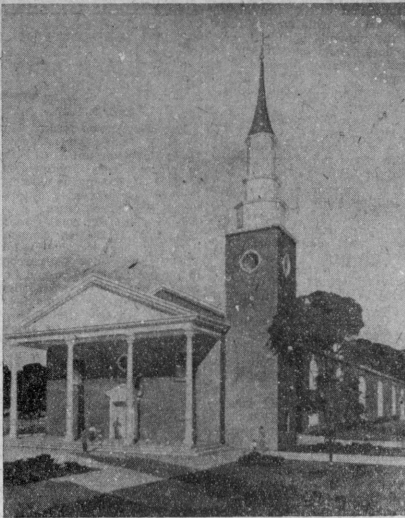
MEMORIAL TO MONSIGNOR GLEISSNER. The new St. Mary's Chapel at College Station, Texas, which is to be a memorial to the late Monsignor J. B. Gleissner, the Aggie Chaplain, is under construction.
