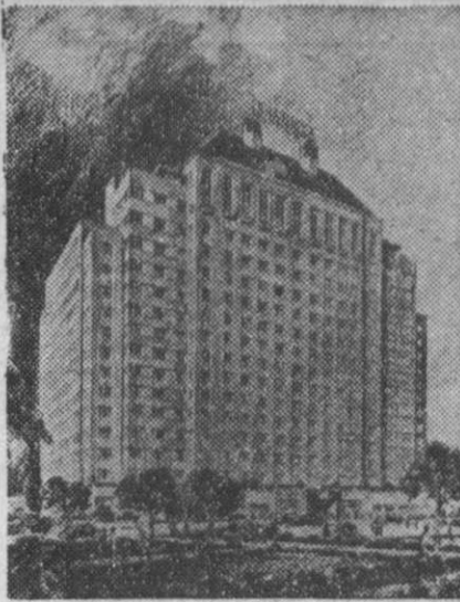
The Shamrock, which opened recently at Houston amid elaborate ceremonies, is America's newest and largest post war hotel. The 18-story Shamrock is the largest steel reinforced concrete structure built since the war. It contains 2,100 tons of steel reinforcing bars and 2,200 tons of structural steel.
